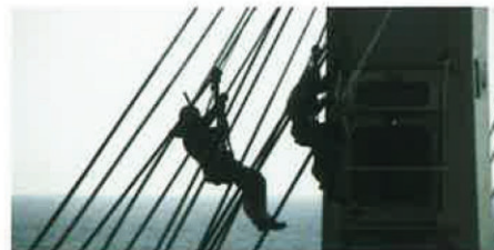
Lara Rickmers - greasing and cosmetic maintenance of deck cranes
