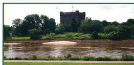
Alter Wasserturm (Old Water Tower)
