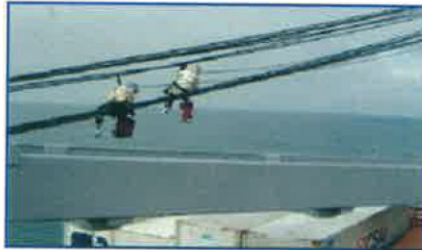
Crane Maintenance onboard M/V "Sea Puma"
