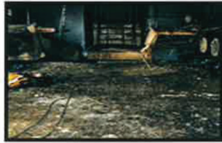
View of engines after fire.
